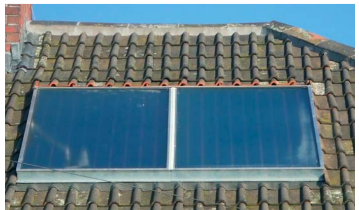
Top: Evacuated-tube solar collector. Bottom: Flat-plate solar collector. (Photographs courtesy of Solar Thermal Ltd)
