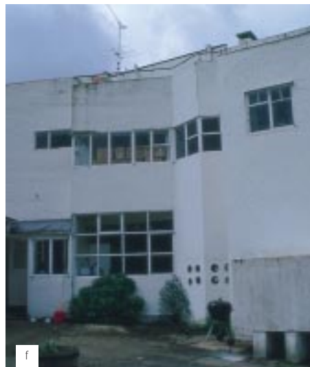
Figure 6 Examples of the wide variety of timber [left] and metal windows [below] found on historic buildings. In (e) the upper part of the frame is metal, the lower part timber. In (f) the thin steel frames of the windows by Crittall are important to the design of this Grade II* Modern Movement building (Connell Ward Lucas, 1932). [Photographs (a), (c) and (d): English Heritage Building Conservation and Research Team; (f) and (i), Chris Wood; (e), (g), and (h) courtesy of Jill Channer, copyright © Jill Channer]
