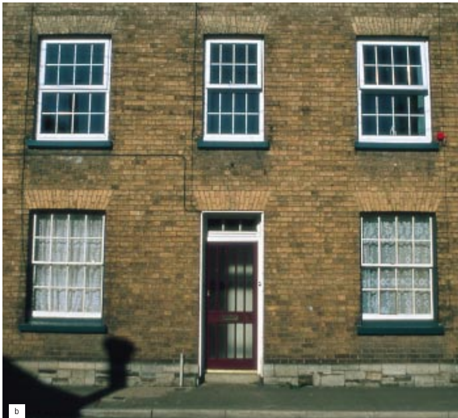
Figure 1 (a, above) Double glazing in PVCu cannot replicate the appearance of an original timber sash with fine glazing bars. (b, right) An unfortunate combination on the same façade: original timber sashes (ground floor), PVCu replacements (first floor) (Photographs: Chris Wood and English Heritage Building Conservation and Research Team)
