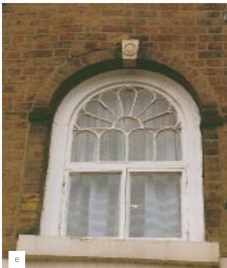
Figure 6 Examples of the wide variety of timber [left] and metal windows [below] found on historic buildings. In (e) the upper part of the frame is metal, the lower part timber. In (f) the thin steel frames of the windows by Crittall are important to the design of this Grade II* Modern Movement building (Connell Ward Lucas, 1932). [Photographs (a), (c) and (d): English Heritage Building Conservation and Research Team; (f) and (i), Chris Wood; (e), (g), and (h) courtesy of Jill Channer, copyright © Jill Channer]
