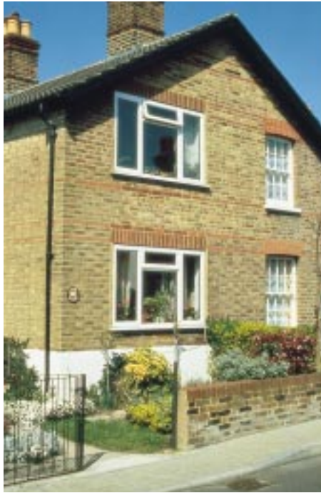
Figure 4 Enlarging the window openings and setting the frames flush with the façade (left) totally distorts the proportion and detailing of the original windows (right). (Photograph courtesy of Kit Wedd)
