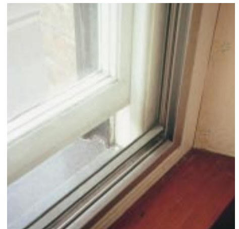
Figure 9 Secondary glazing can provide very effective thermal improvement. In historic buildings its successful insertion depends on fitting within the reveal in such a way as not to damage historic fabric. However, secondary glazing can sometimes produce an unsatisfactory reflection when viewed from the outside. (Photograph courtesy of Kit Wedd)
