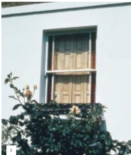
Figure 4 Enlarging the window openings and setting the frames flush with the façade (left) totally distorts the proportion and detailing of the original windows (right). (Photograph courtesy of Kit Wedd)
