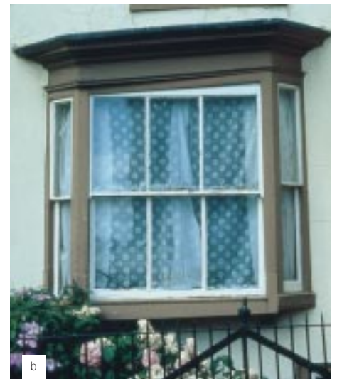
Figure 5 Historic glass, especially Crown glass, is rare and cannot be reproduced today. Where examples such as the middle right pane survive, they must be preserved. (Photograph courtesy of Treve Rosoman)
