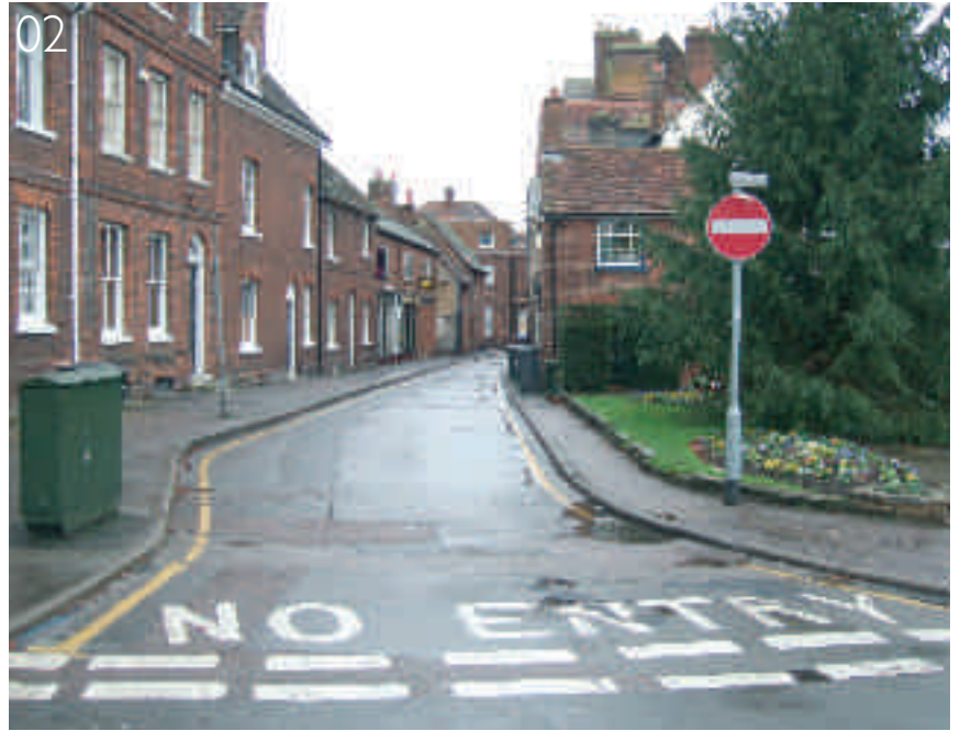
02 An excess of signing – the overall design should remove the need for this through better road alignment and sign location
