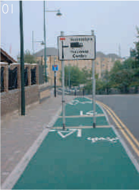
01 Over elaborate signing implemented without any thought to its location and the impact it has on the street environment and the confusion of message it gives
